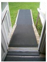
A threshold may not be higher than  $\frac{3}{4}$ " in existing construction. A tapered transition strip will reduce the trip hazard at this threshold. The upper ramp landing must be at the same level as the interior floor.
