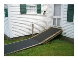
Landings at top and bottom must be level: the bottom landing must be at least as wide as the ramp. At the top, maneuvering space is required at the doorway, so the landing must be at least 60" deep, perpendicular to the door, and allow at least 18" clear space on the latch side of the door to provide a visitor sufficient room to maneuver past the out-swinging door.
